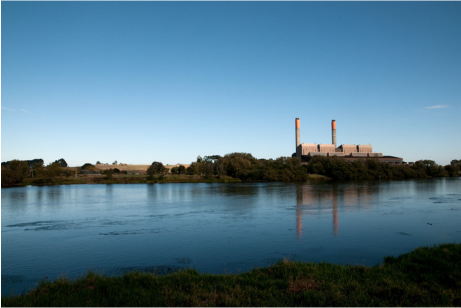
Genesis' Huntly Power Station.
