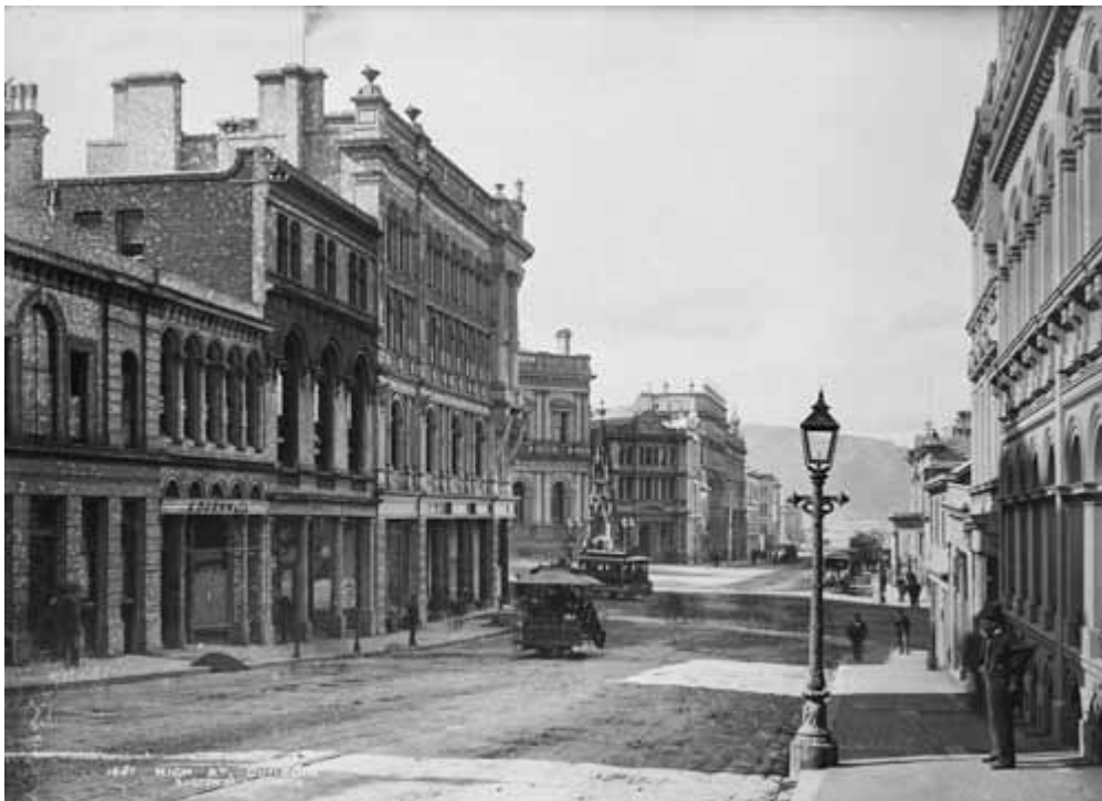
Watsons' Commercial Hotel, built in 1874 by John and James Watson on High Street in Dunedin, is the brick building with three storeys on the left near the trolley. In 1878, a regular customer estimated that they had a lunchtime rush of 400 people per day. C.012093, Museum of New Zealand Te Papa Tongarewa.
